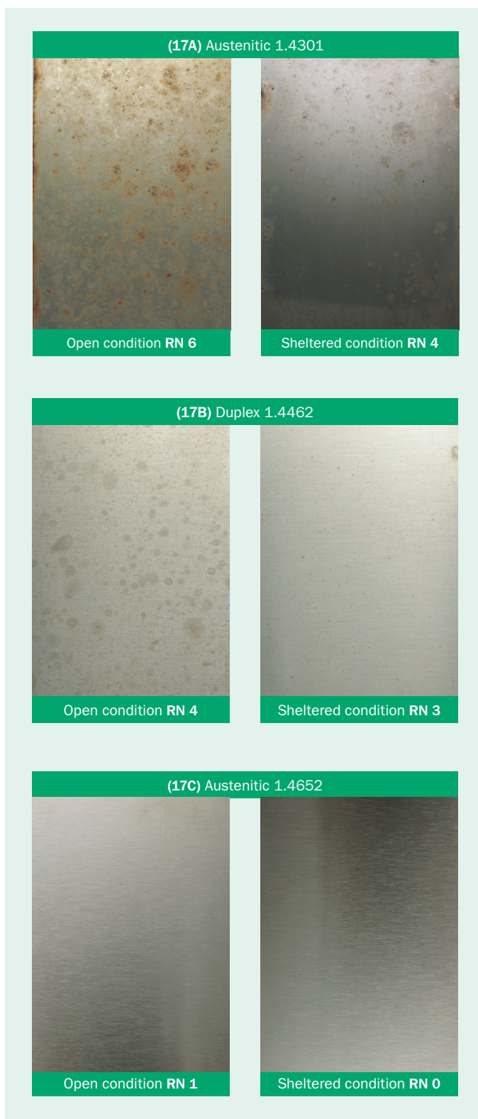
Figure 17 Appearance of stainless steel surface after 4 years exposure with different exposed condition
