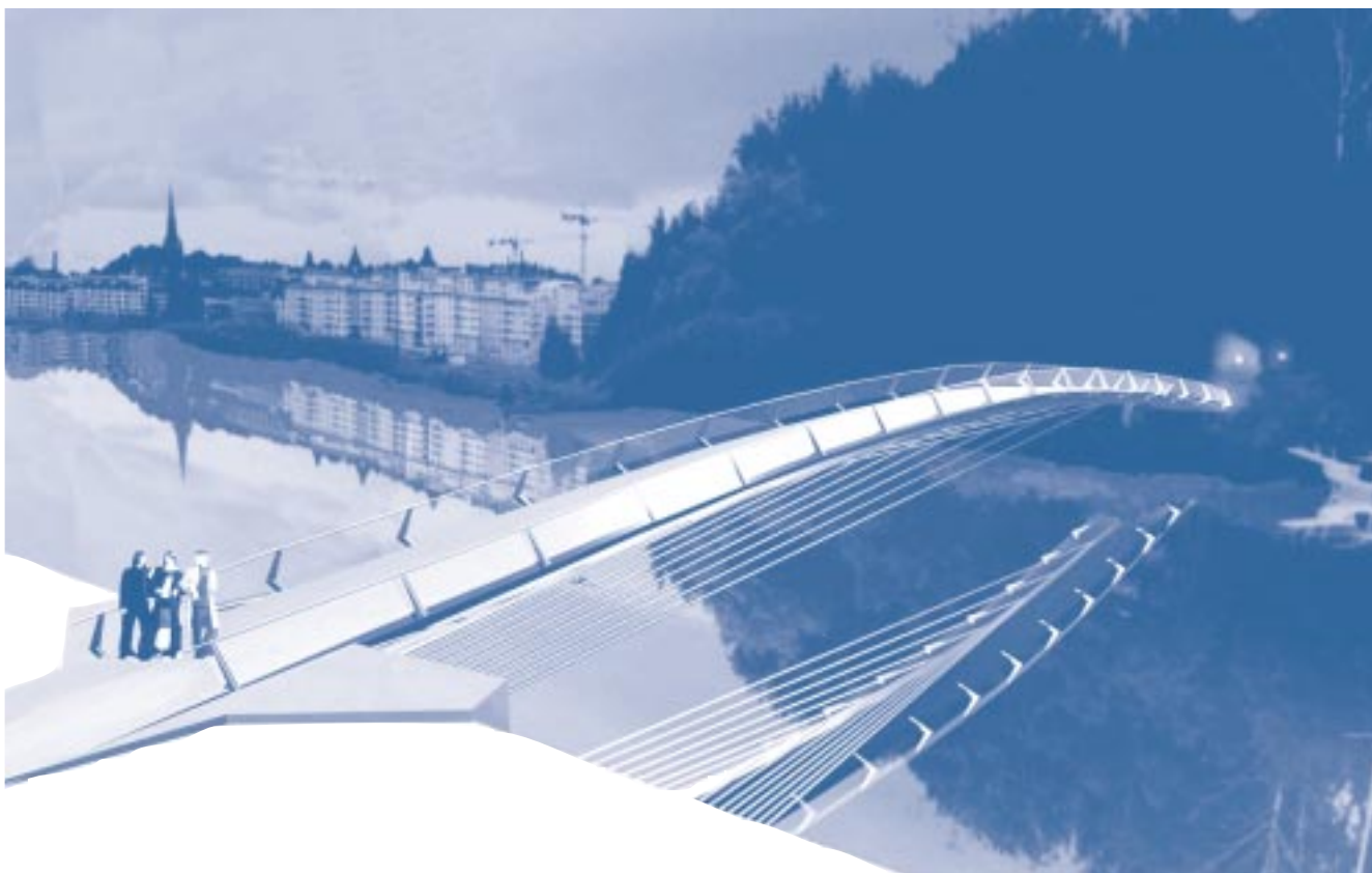
Figure 5: The Apaté-bridge at Sickla channel in the centre of Stockholm. Bridge made of DSS (1.4462) under construction. (Created by Magnus Ståhl & Erik Andersson)
