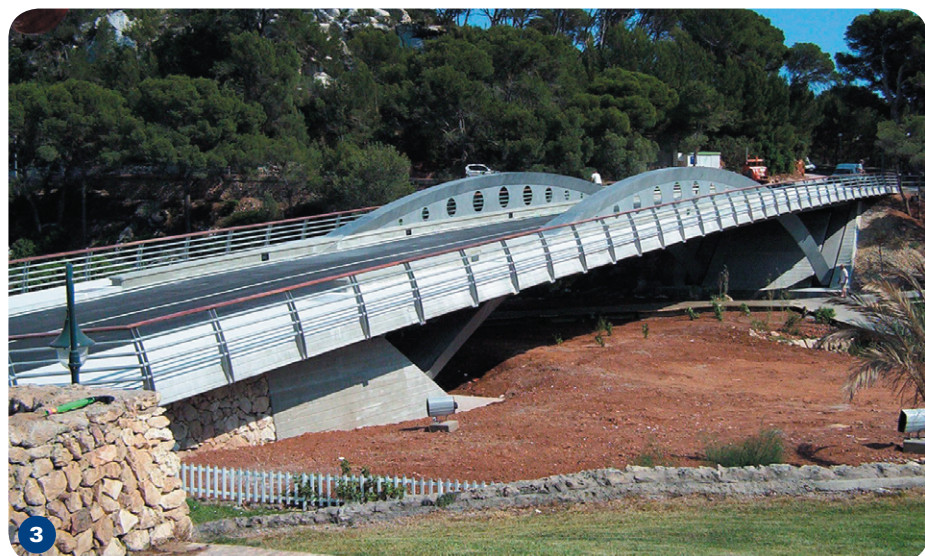
Fig. 11 Bridges made of LDX 2101 (1), 2304 (2) and 2205 (3).
