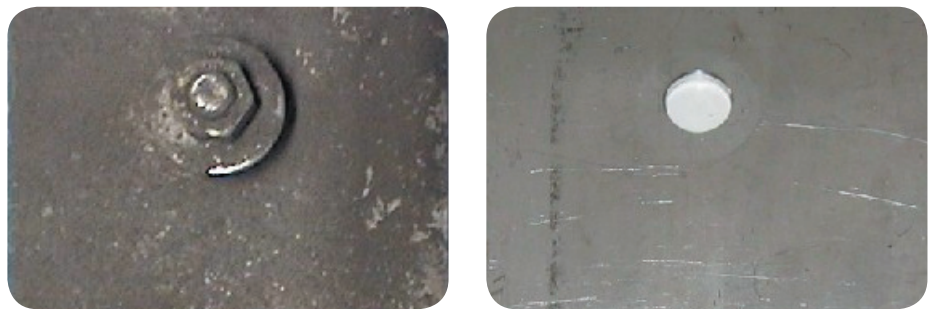
Fig. 8 Specimens made of 316L after 4 years in the Söderledstunnel before (left) and after cleaning.
