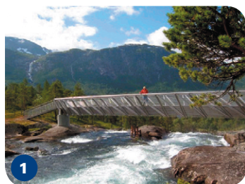
Fig. 11 Bridges made of LDX 2101 (1), 2304 (2) and 2205 (3).
