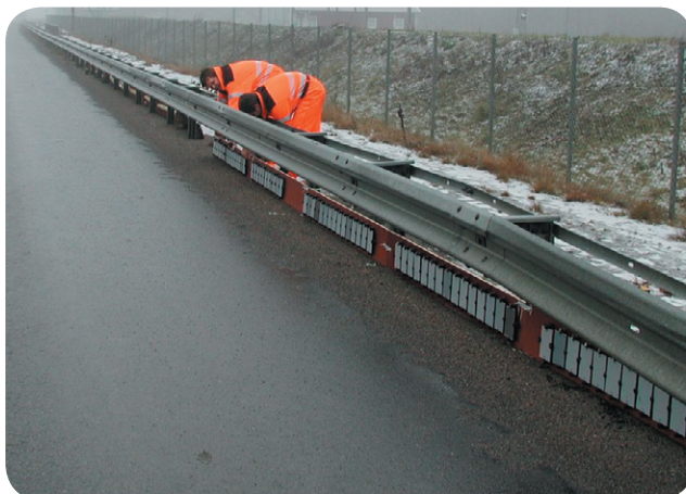
Fig. 3 Plyfa sheets with specimens, Borås (left) and the Öresund bridge (right).
