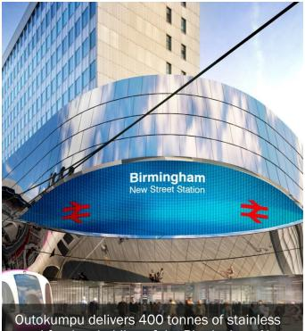
Outokumpu delivers 400 tonnes of stainless steel for the cladding of the Birmingham New Street station in the UK. More than 8,000 bright-polished, lasercut panels will cover the façade.
